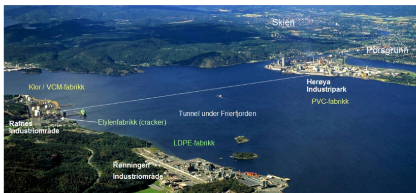
Figure 6. By-product hydrogen from INOVYN's VCM-factory at Rafnes being fed through a tunnel underneath the Frierfjord supplying the Porsgrunn refuelling station with FC-grade hydrogen (Blue Move, 2018).
